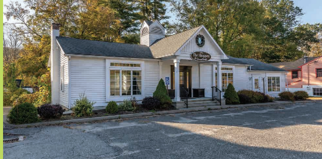
Prime 2 Unit Retail/Commercial Building. 2 Half Baths. Excellent Storage. Large Parking Area. 2,000+ Cars Per Day. 0.22± Acres. $399,000. Graham Klemm. 860.868.7313.
