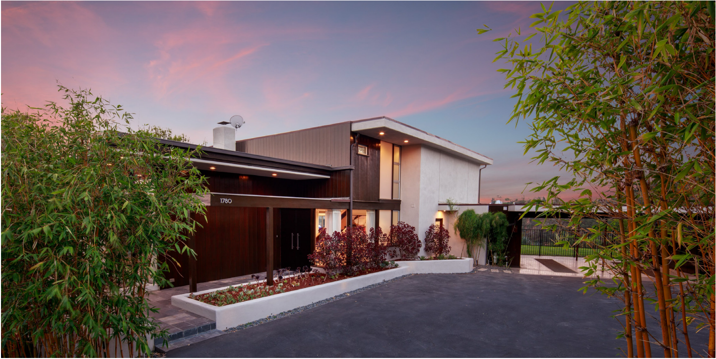
11780 STONE CANYON ROAD LOS ANGELES, CALIFORNIA
