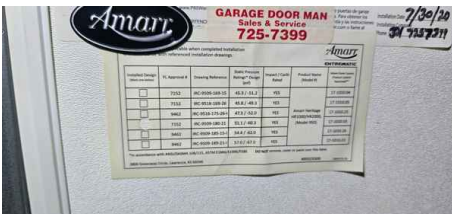
Large missile impact rated labels for non-glazed garage doors
