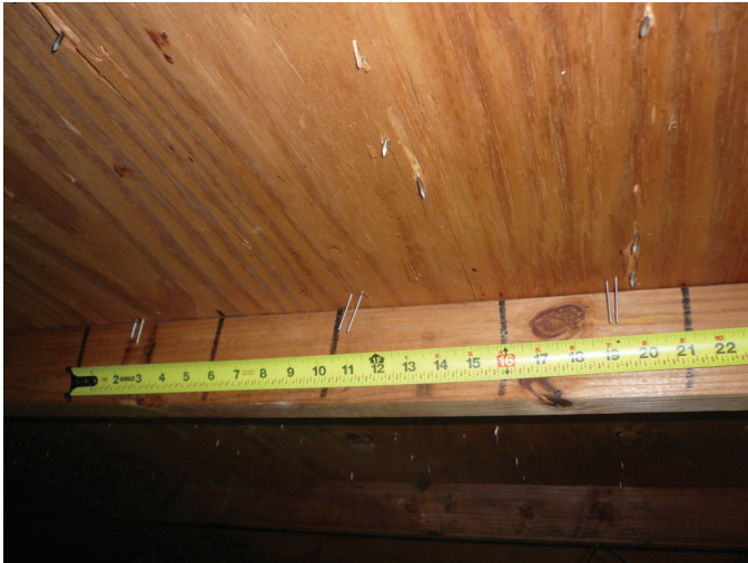
8d nails on 6" spacing
