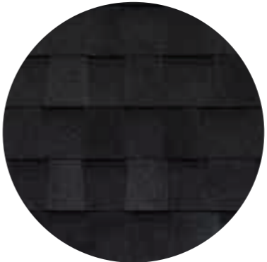
Black shingle roof
