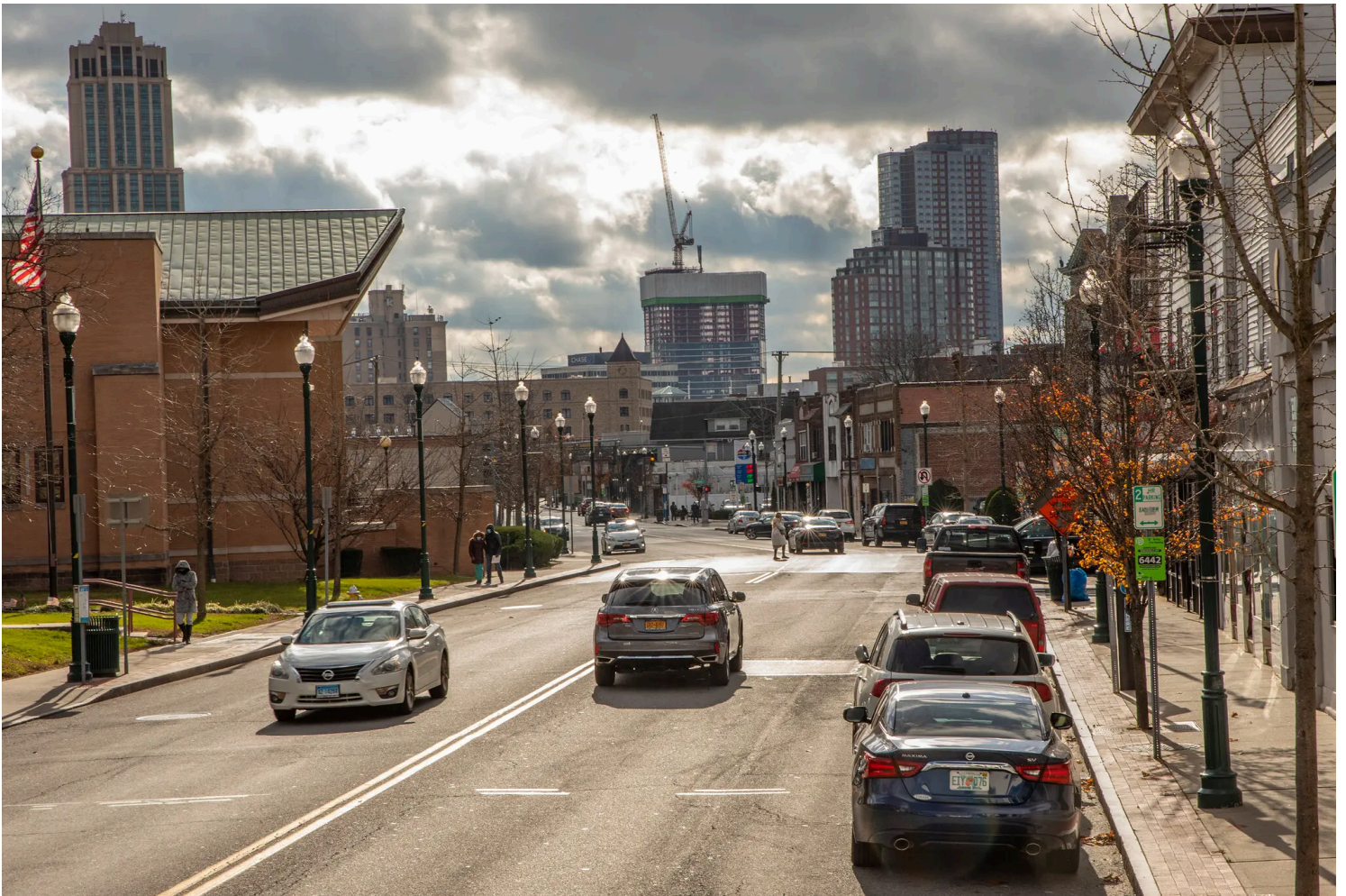
North Avenue, looking toward downtown, where 10 towers, all rental buildings, are under construction. Tony Cenicola/The New York Times
