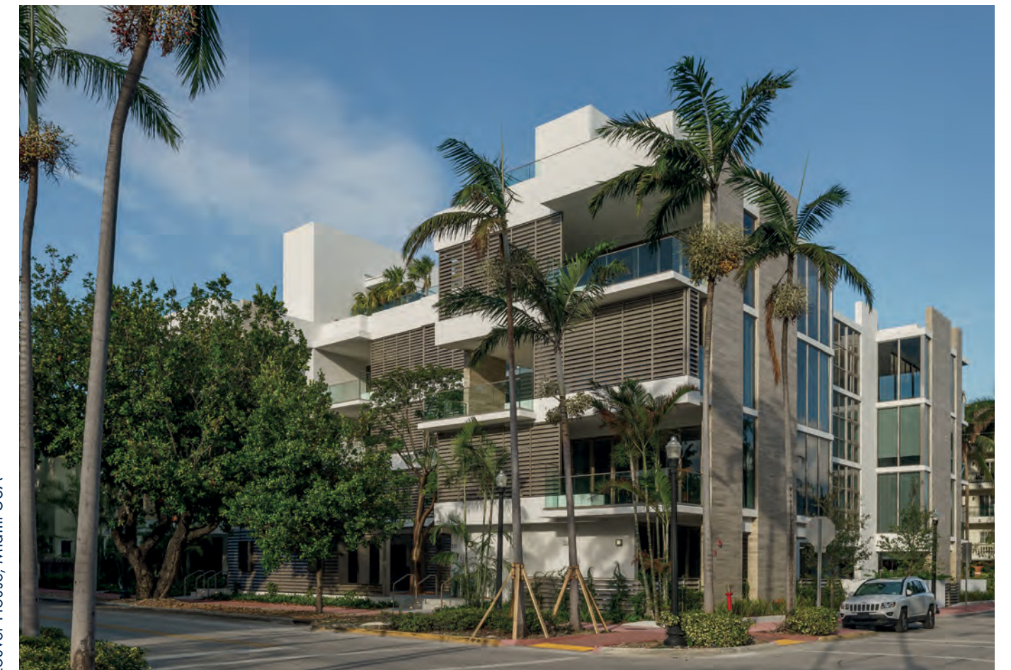
Louver House, Miami USA
