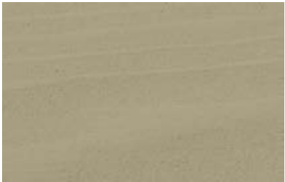
Ceiling Stain Direction
