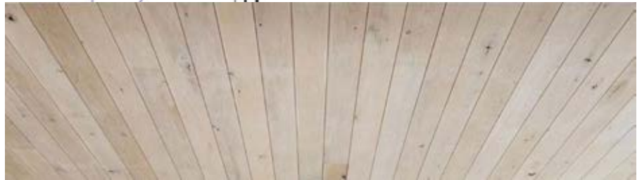
Plank Ceiling Painted
