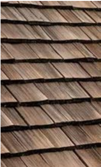
Wood Shake Roof
