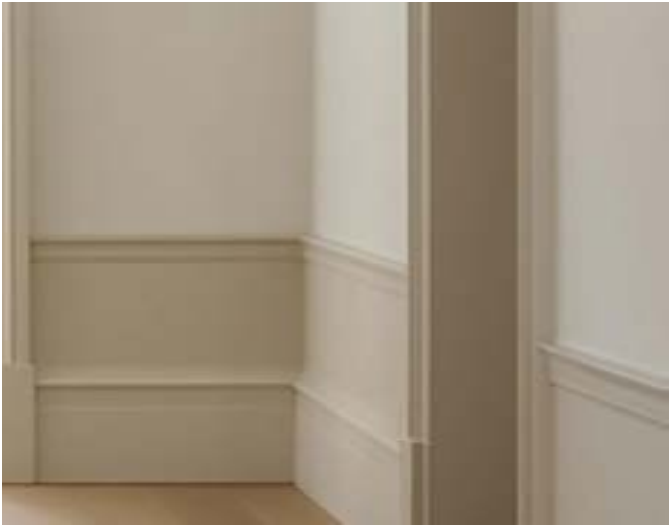
Baseboard Trim Painted
