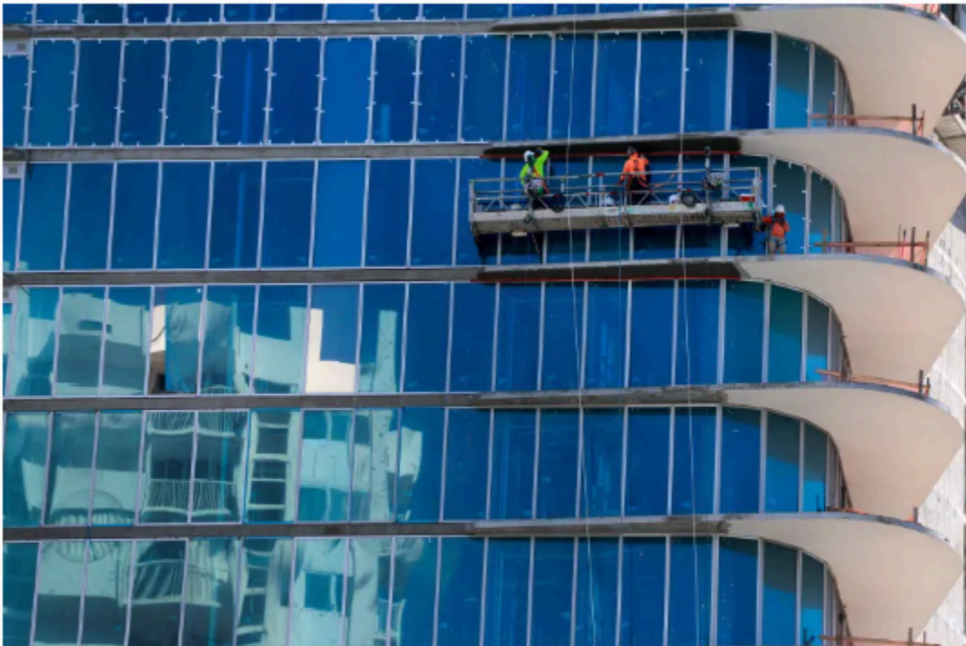
(Mike Stocker/South Florida Sun Sentinel) The Ritz Carlton on State Road A1A in Pompano Beach under construction on Feb. 26, 2025, is part of the development initiatives occurring in Pompano Beach. (Mike Stocker/South Florida Sun Sentinel)
