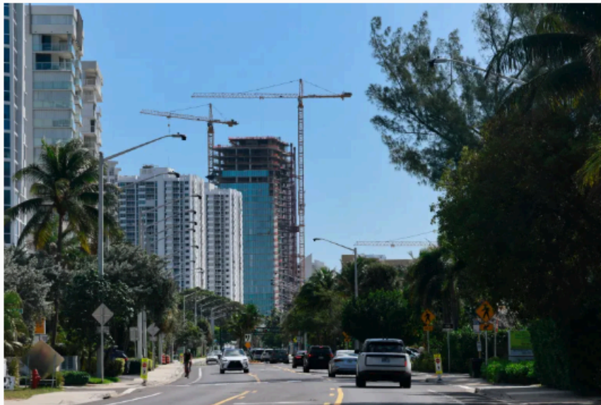
(Mike Stocker/South Florida Sun Sentinel) The Ritz-Carlton Residences on South Ocean Boulevard in Pompano Beach is shown under construction on Feb. 26, 2025. The project's construction is one of the many changes underway. (Mike Stocker/South Florida Sun Sentinel)
