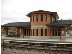
Dee Road Station 881 North Dee Road, Park Ridge
