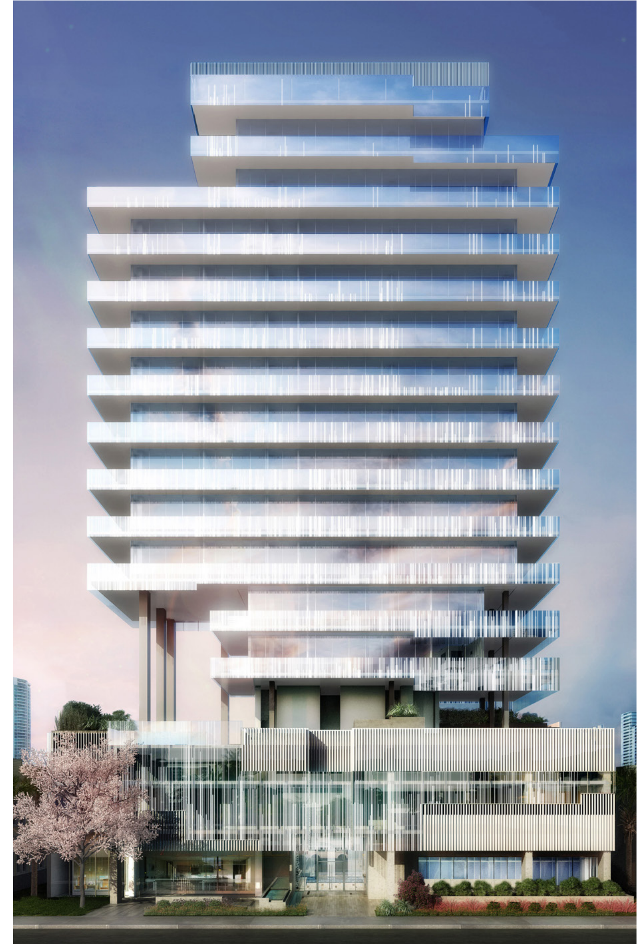
DESIGNED BY ARCHITECT RENE GONZALEZ, TERRA GROUP'S 18-STORY GLASS RESIDENTIAL TOWER USES TRANSPARENCY TO BLEND INTO THE MIAMI BEACH LANDSCAPE.
