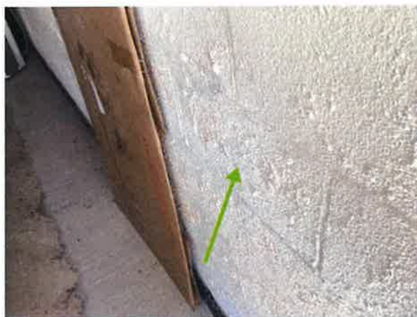
Efflorescence
