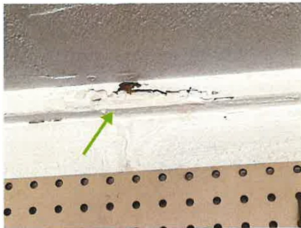
Garage back wall
