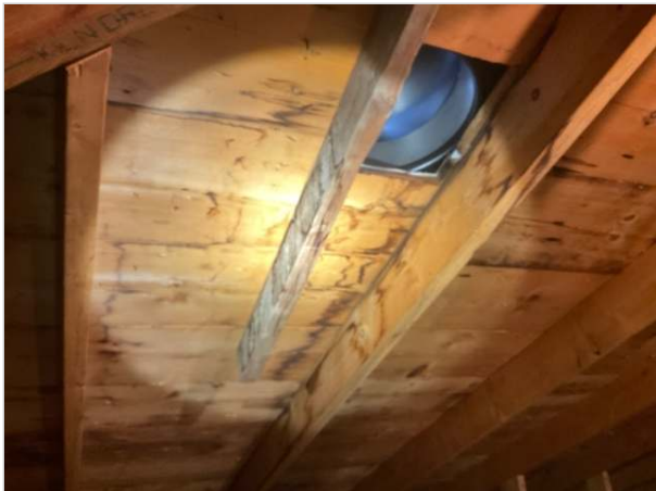
examples of watermarked roof decking. All accessible watermarks were dry at the time of inspection
