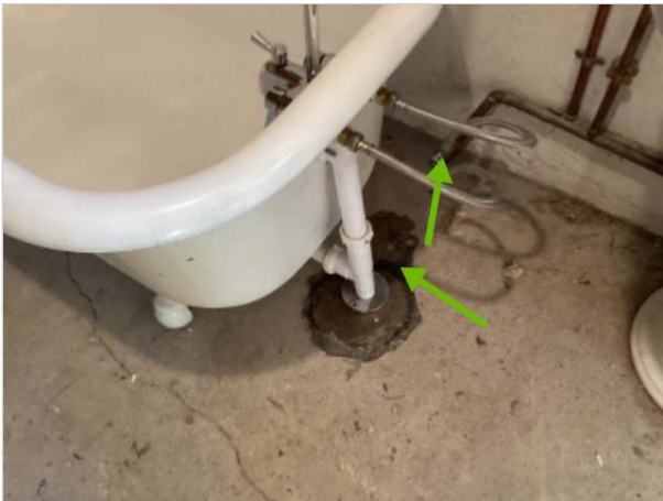
Valve leak
