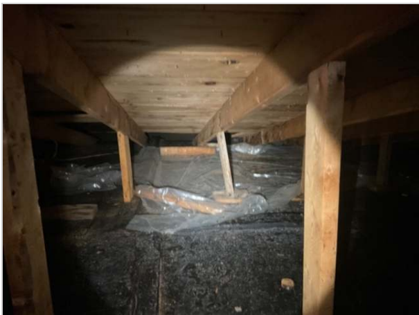
examples of questionable and out of plumb support
