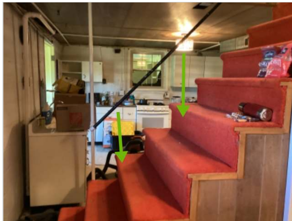
Recommend vertical balusters
