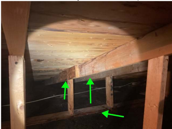
examples of watermarked roof decking. All accessible watermarks were dry at the time of inspection
