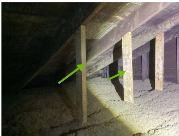
Evidence of previous adequate reinforcement
