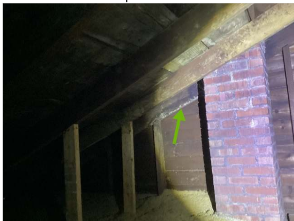
Recommend upgrading ventilation at next roof replacement
