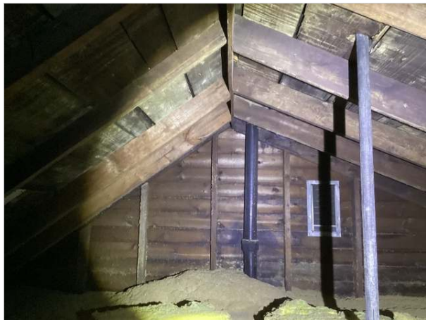
Recommend upgrading ventilation at next roof replacement
