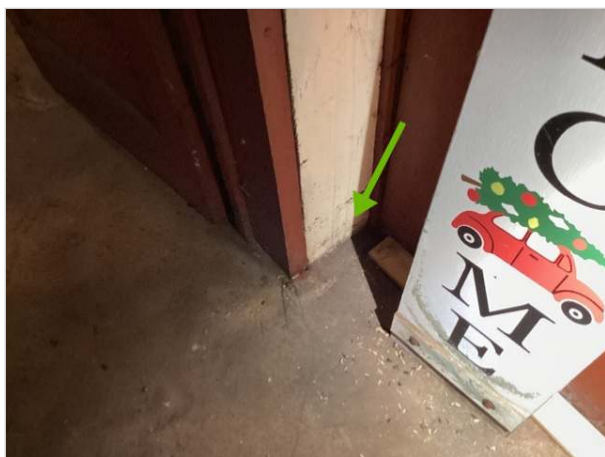
Under front porch
