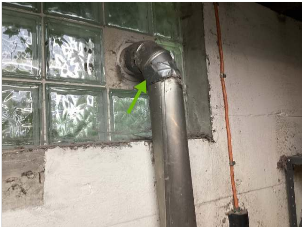
Recommend foil tape versus duct tape
