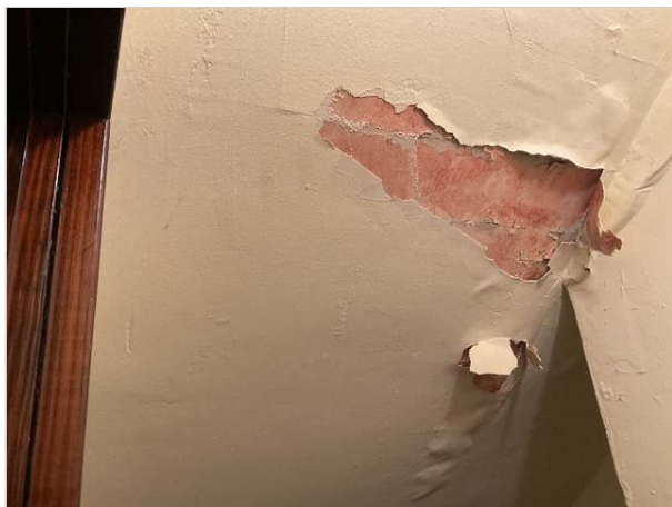
front bedroom closet
