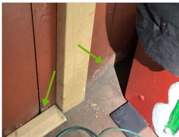
Under front porch
