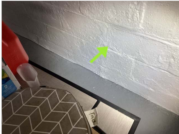
Under front porch
