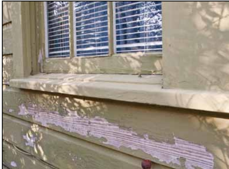
TEXAS CASE LAW addressing “as-is” agreements in residential transactions has revolved around everything from leaking roofs, defective foundations, faulty plumbing and air conditioning to electrical wiring.
