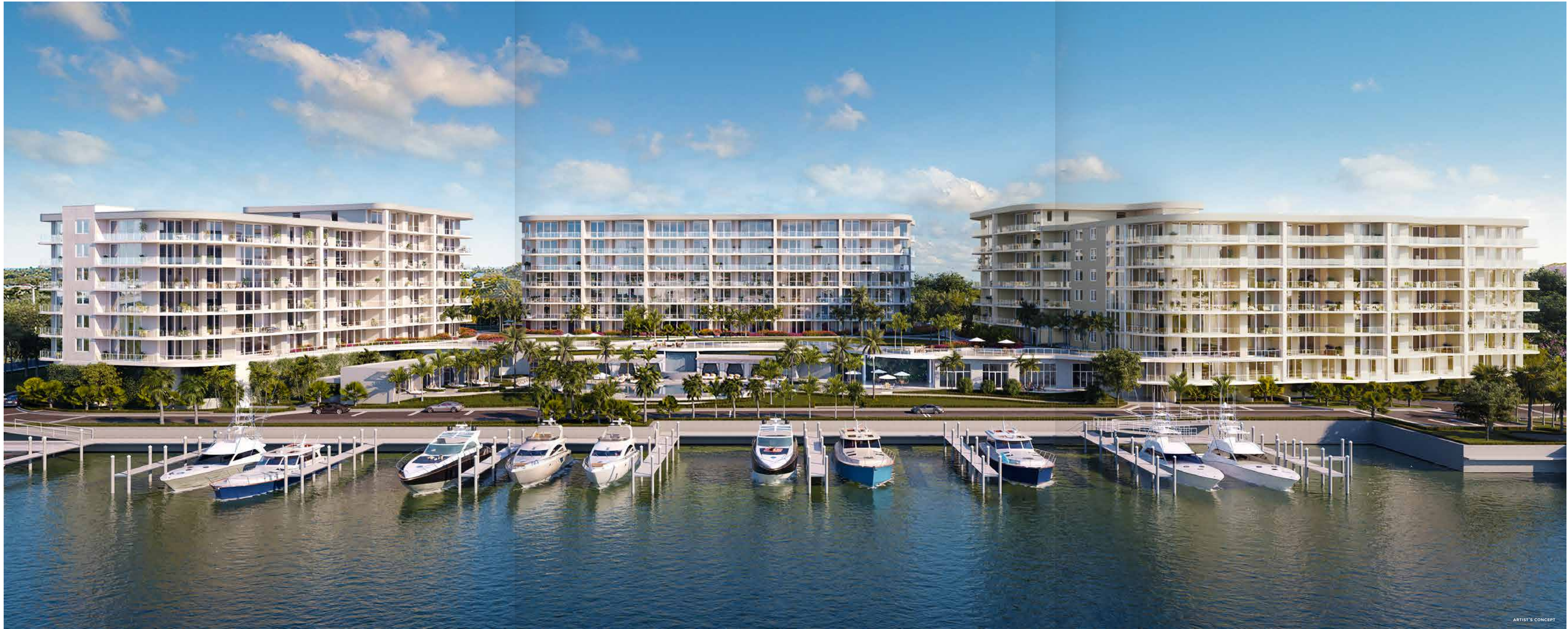
The Residences feature three, seven-story residential buildings across fourteen acres of Palm Beach Gardens' most pristine stretch of Intracoastal waterfront.
