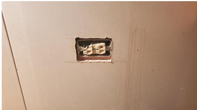
Basement sink outlet
