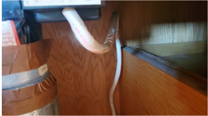
Unprotected wiring
