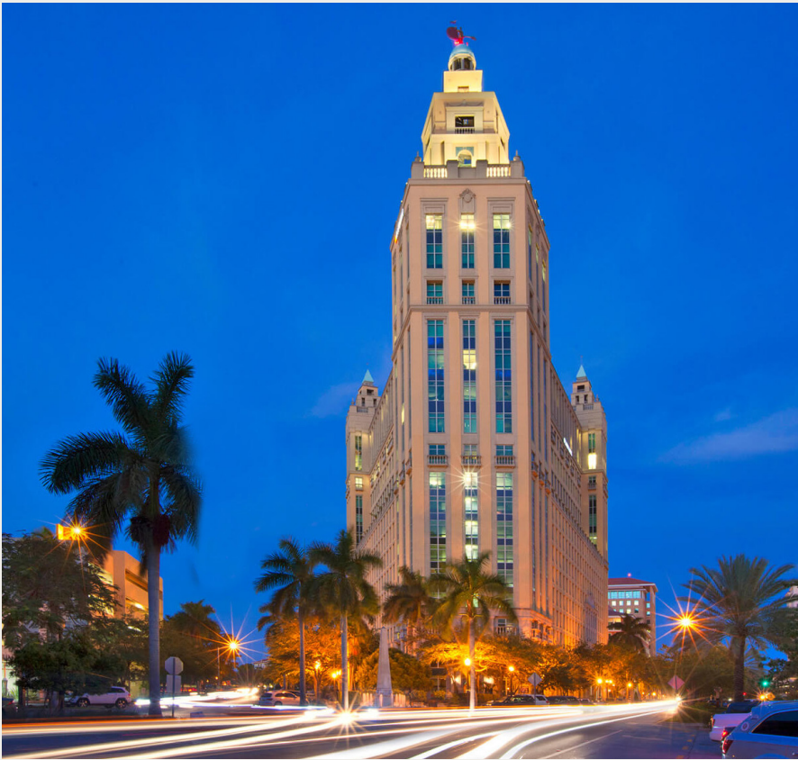
Alhambra Towers, Coral Gables, FL
