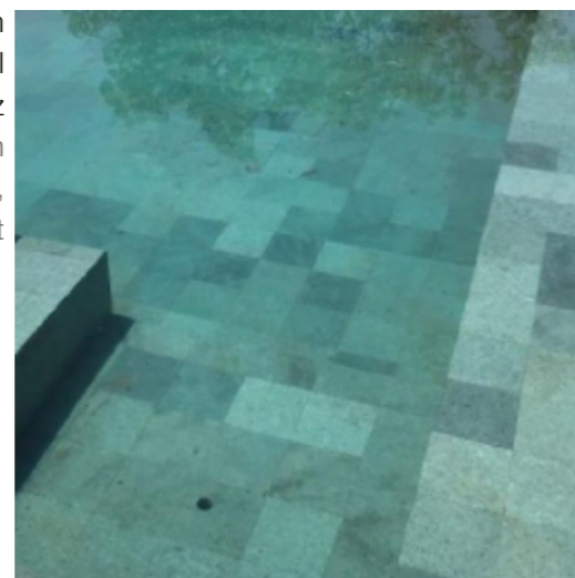
Pedra verde tailandia com estereotomia desencontrada Thailand green stone with stereotomy mismatched
