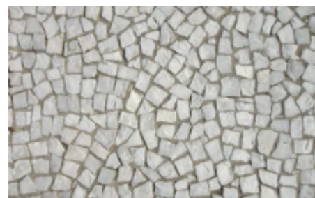
Pedra de calçada 5x5cm na rua Paving Stone 5x5cm on the street
