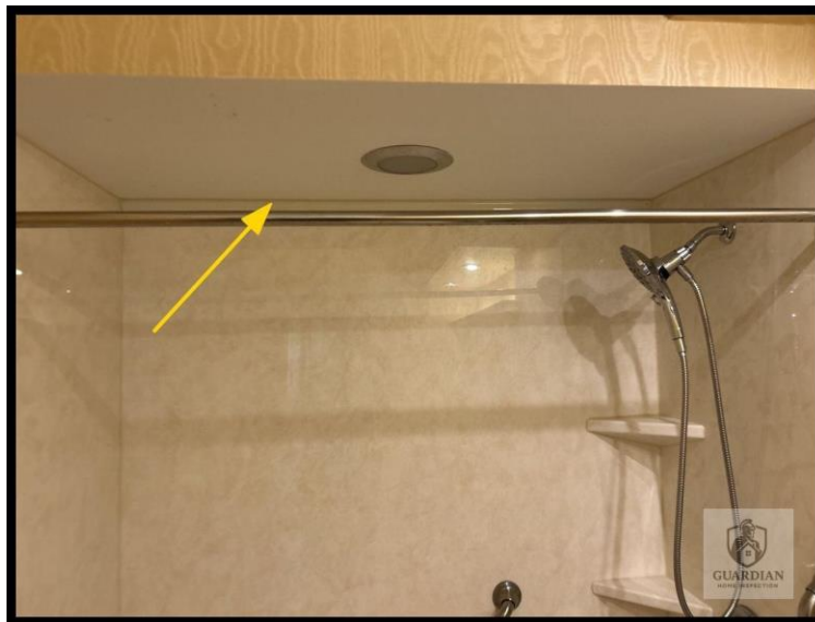
Figure 6: Several light bulbs were observed to be blown/non-functional at light fixtures in the living room, bathroom, and kitchen.
