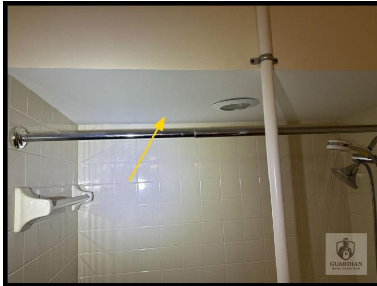
Figure 5: Several light bulbs were observed to be blown/non-functional at light fixtures in the living room, bathroom, and kitchen.
