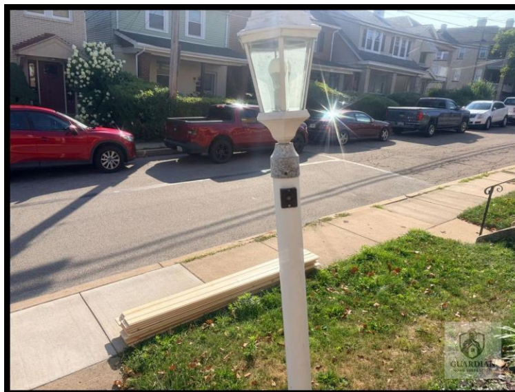
Figure 12: An exterior lamp post was observed to be loose/unstable.
