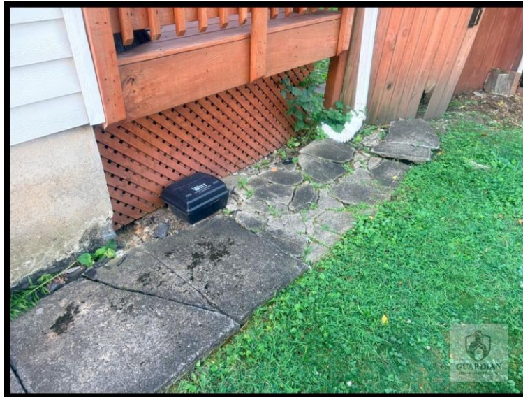
Figure 5: Cracked and broken concrete was observed at the exterior walkway/landing, with vegetation growth through the damaged areas and resulting uneven surfaces.
