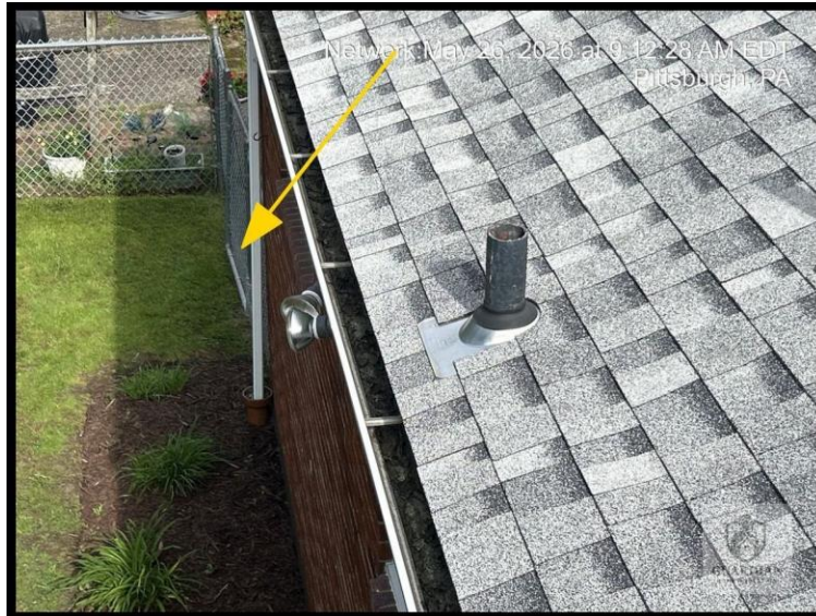
Figure 13: Debris was observed accumulated in the gutters at the roofline.
