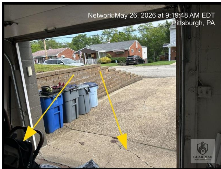
Figure 20: The garage door opener would only close when the wall control button was held down, which commonly indicates a fault or misalignment with the photoelectric safety sensors.
