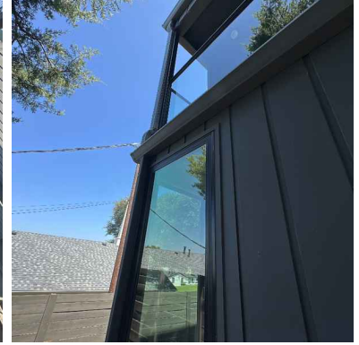
Top of window trim
