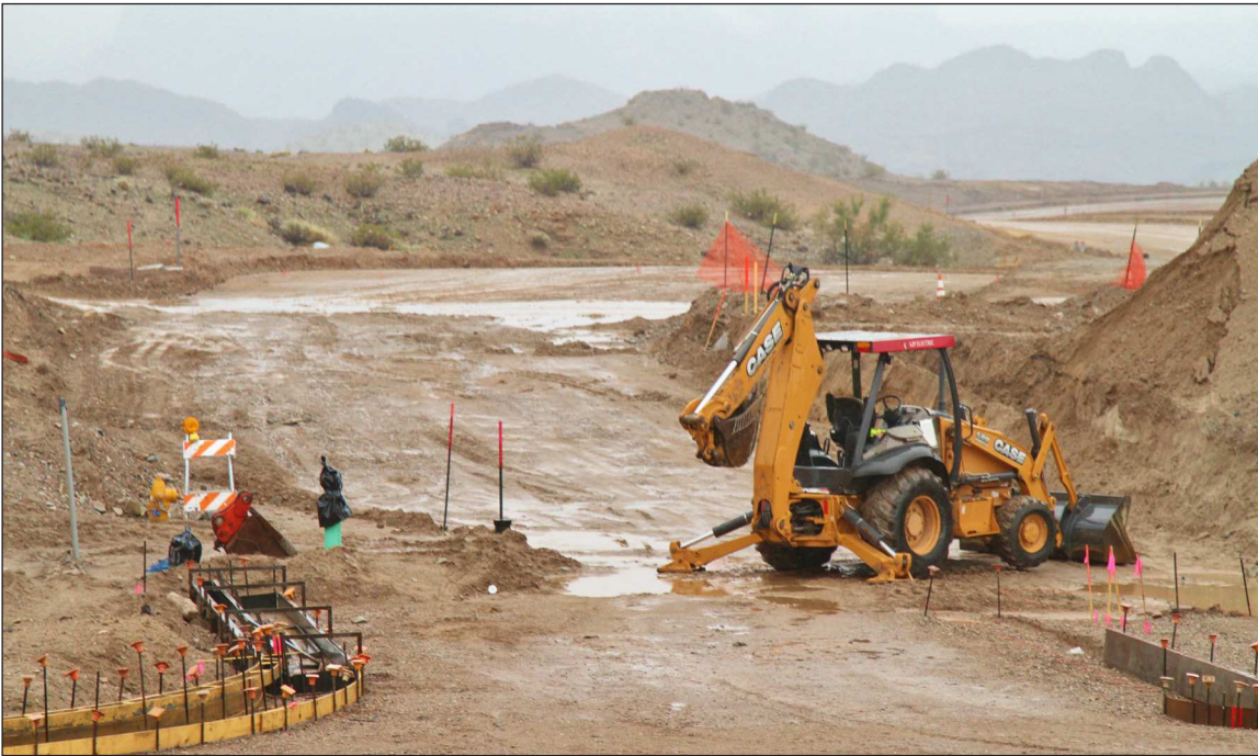
Brandon Messick/Today's News-Herald The Havasu Riviera Parkway nears completion, according to city officials, and is expected to finish construction by mid-March.
