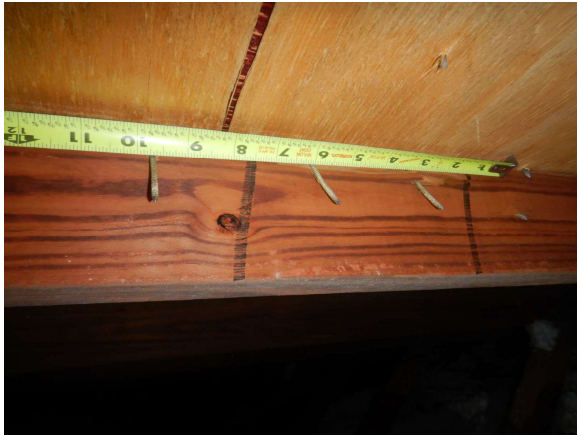
Roof Deck Attachments – 6 Inch in Field
