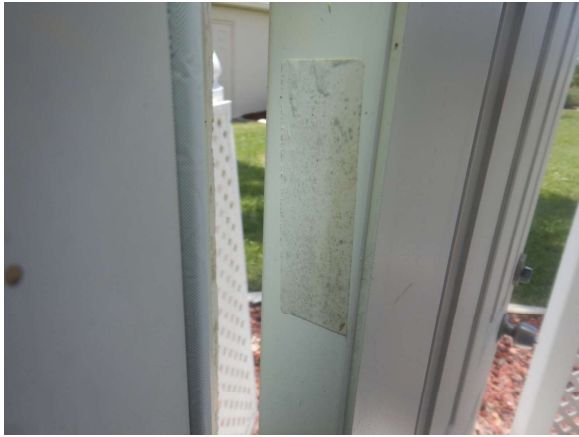
Protection Systems – Storm Impact Door (data tag faded) (Out swinging door with metal skin both sides)
