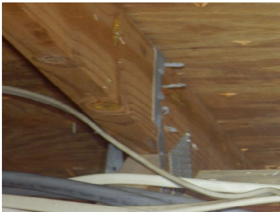
Roof to Wall Attachments – Straps
