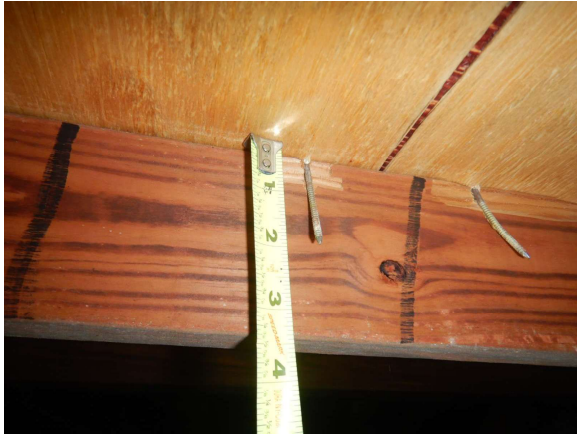
Deck Attachments – 8d Nails
