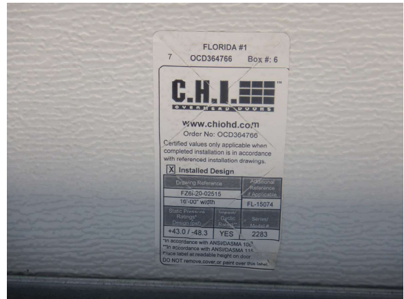
Protection Systems – Garage Bracing & Impact
