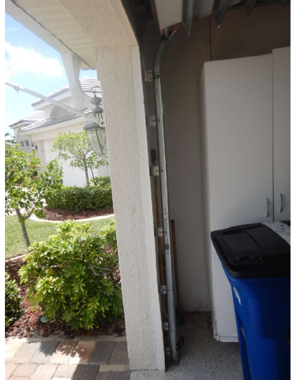
Protection Systems – Garage Bracing & Impact
