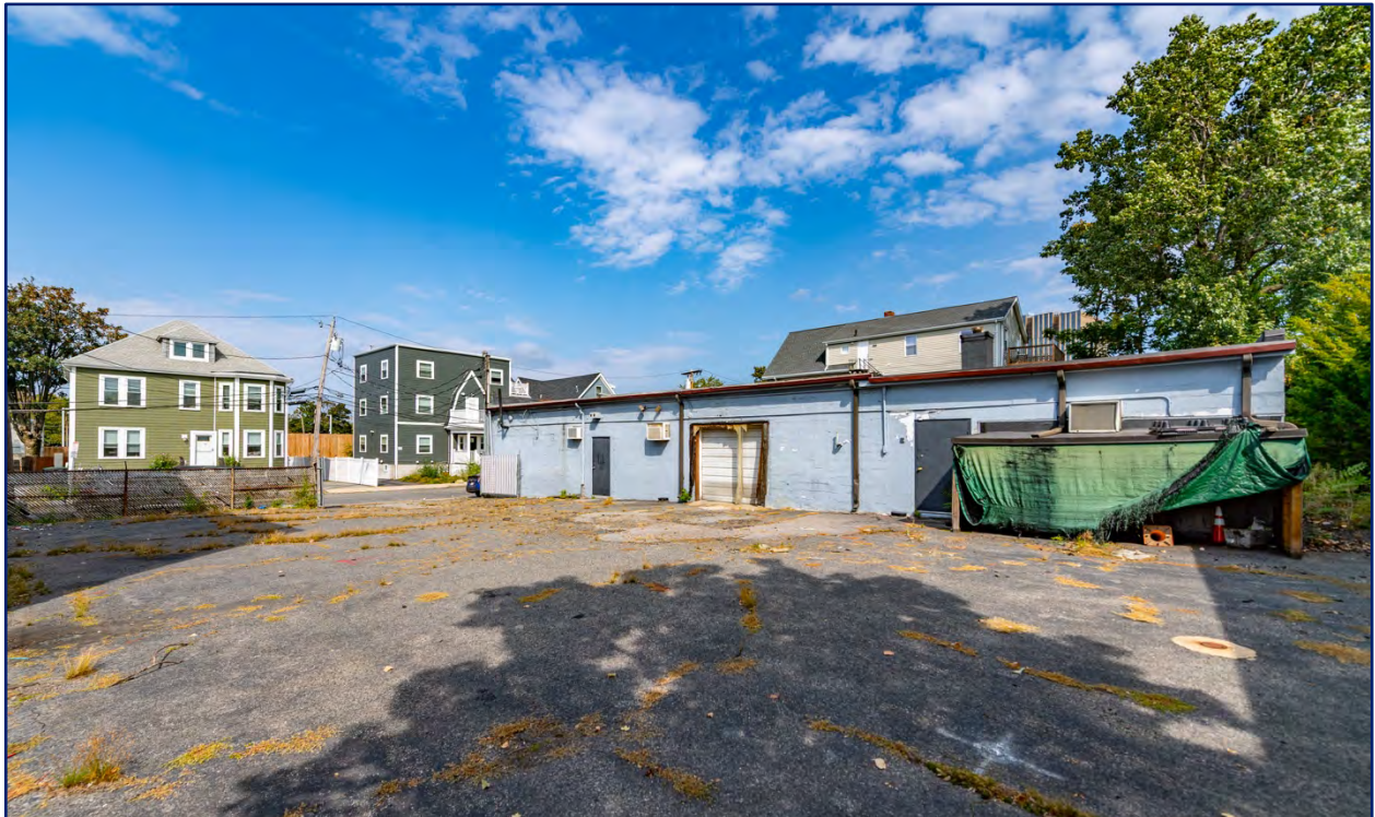
View of the existing building and parking lot
