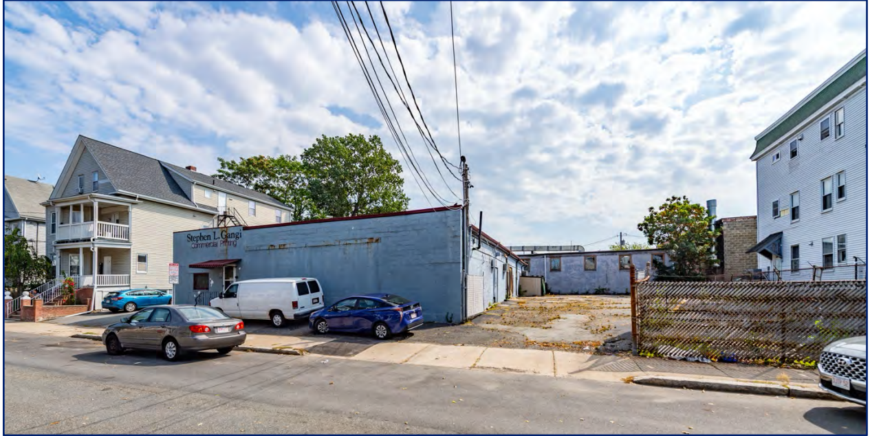
17 Kensington Avenue view from the street
