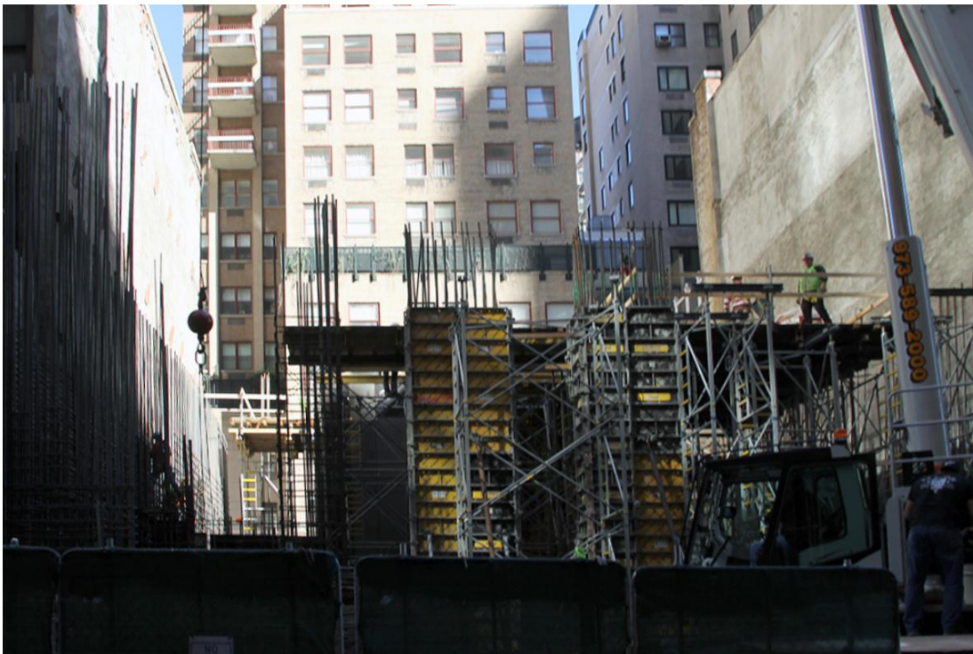
The construction site as of this week, via CityRealty
