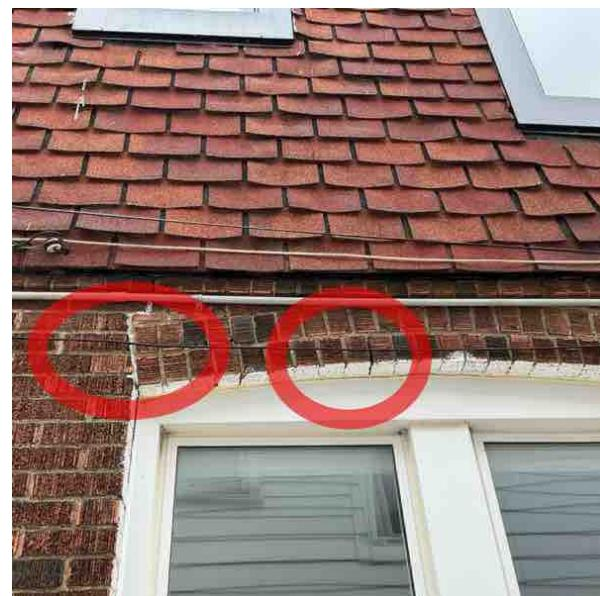
3.4.2 Typical step cracking noted. Recommend repointing or sealing to prevent further deterioration.
