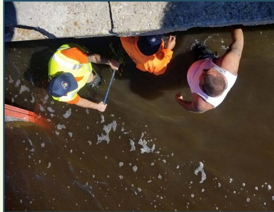
OF-0142 (After): completing valve installation
