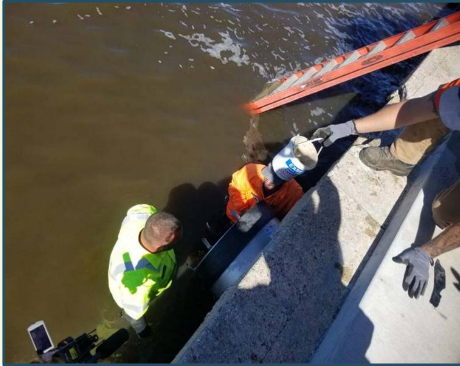
OF-0142 (After): valve inserted into outfall pipe
