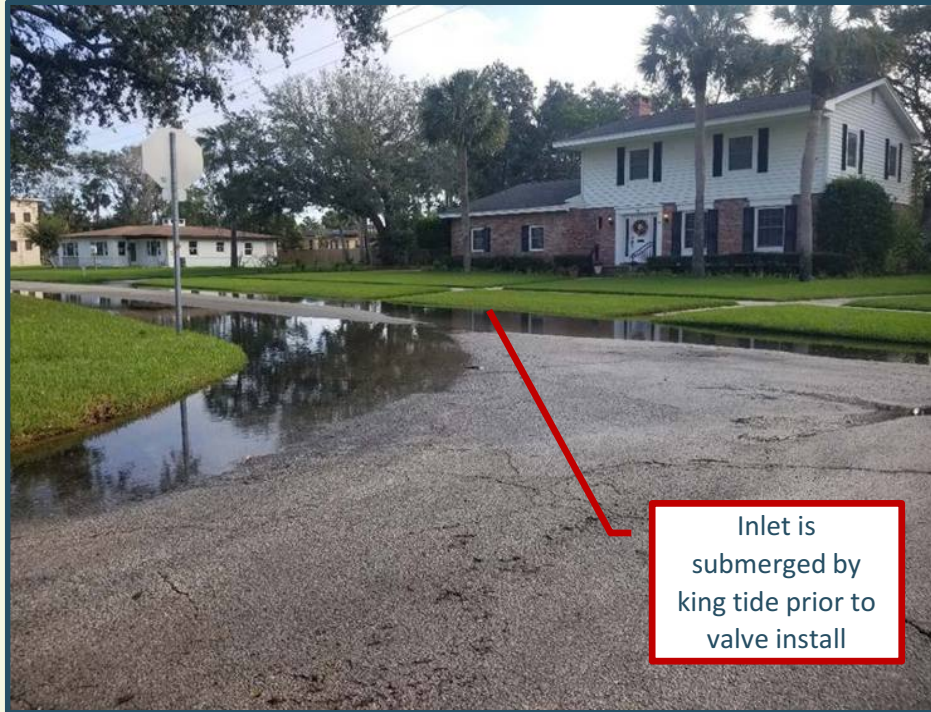
OF-0142 (Before): street flooding during King Tide event (October 2017) due to no valve in outfall
