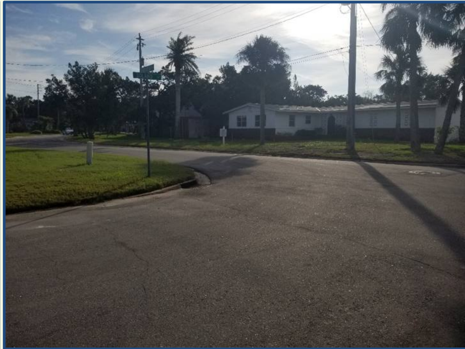
OF-0117 (After): no street flooding during King Tide event (December 2017) - tidal flooding eliminated
