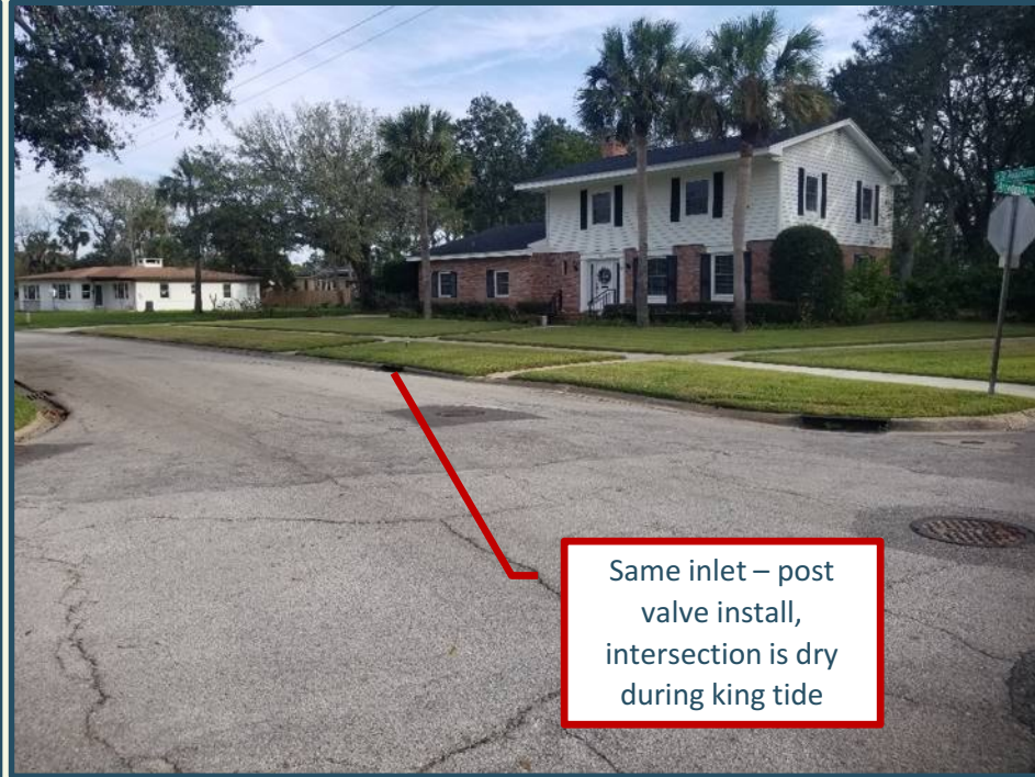
OF-0142 (After): no street flooding during King Tide event (December 2017) - tidal flooding eliminated
