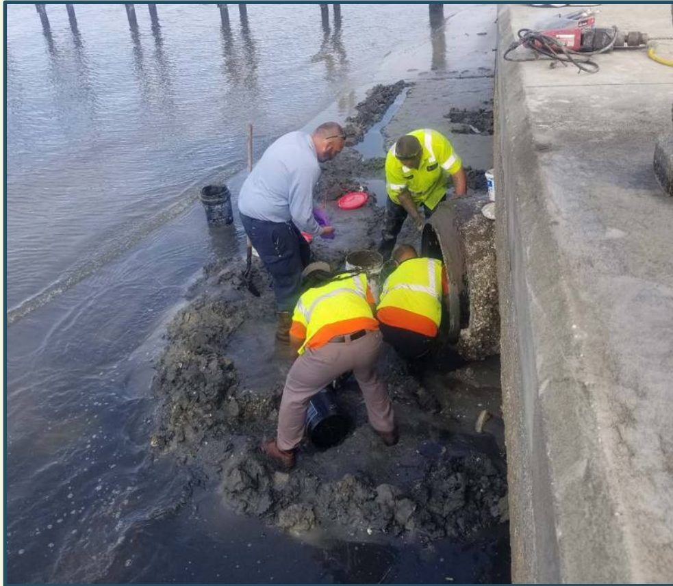
OF-0142 (After): Crew installing valve into outfall pipe
