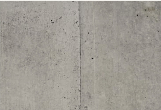
LOWER LEVEL WALLS Exposed Concrete
