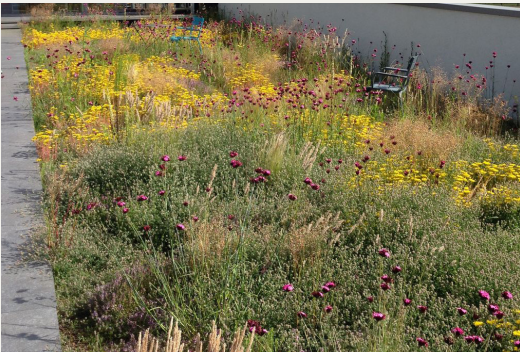
VISIBLE LOW-SLOPE ROOFS Green Roof
