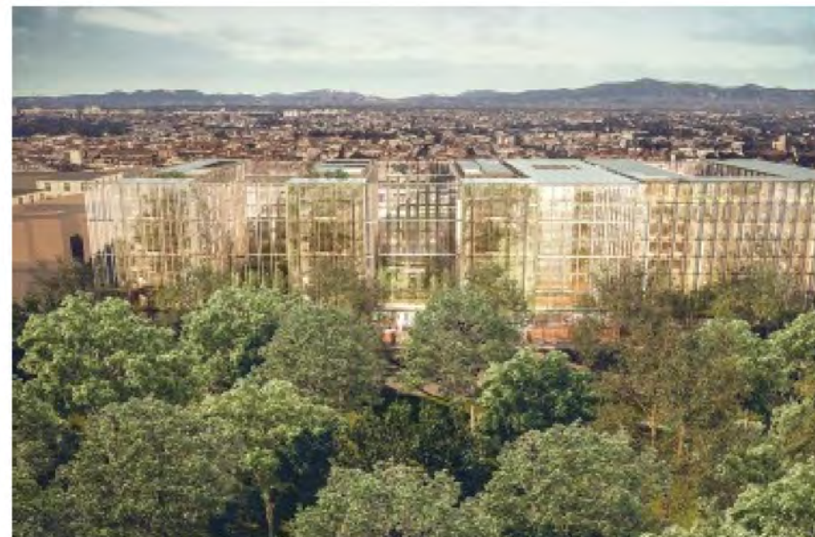
ENEL HEADQUARTERS ROME
