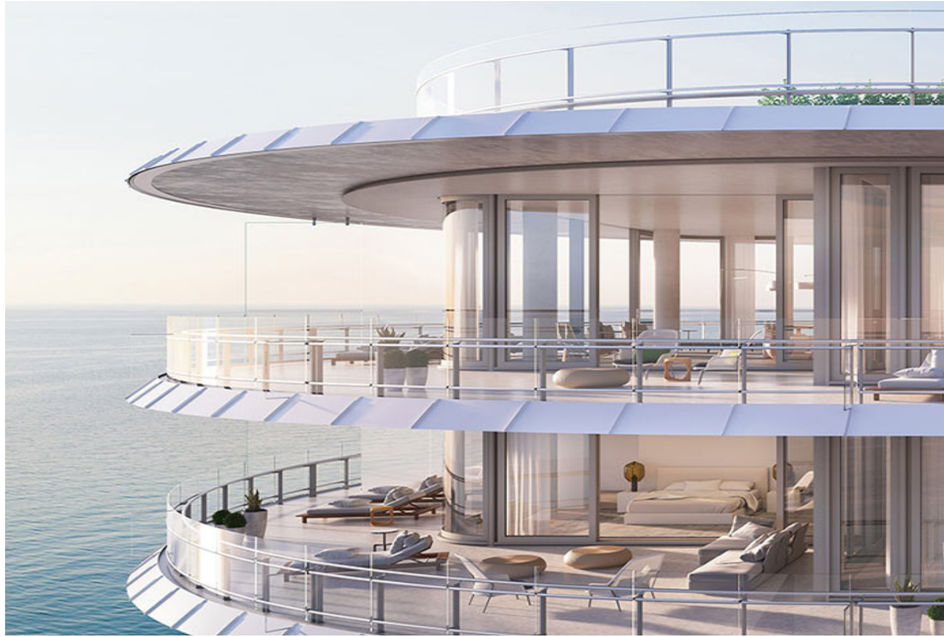
Eighty Seven Park This beachfront condominium is the first residential building designed by Renzo Piano.
