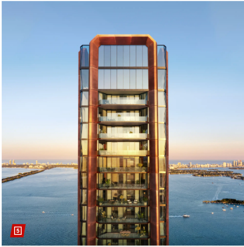
Villa Miami will be 58 stories high when completed in 2026. Binyan Studios
