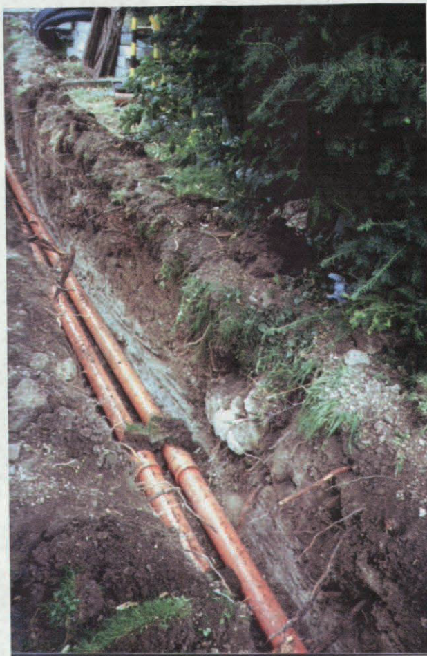
Plate 9: Watching brief: Wall footing
