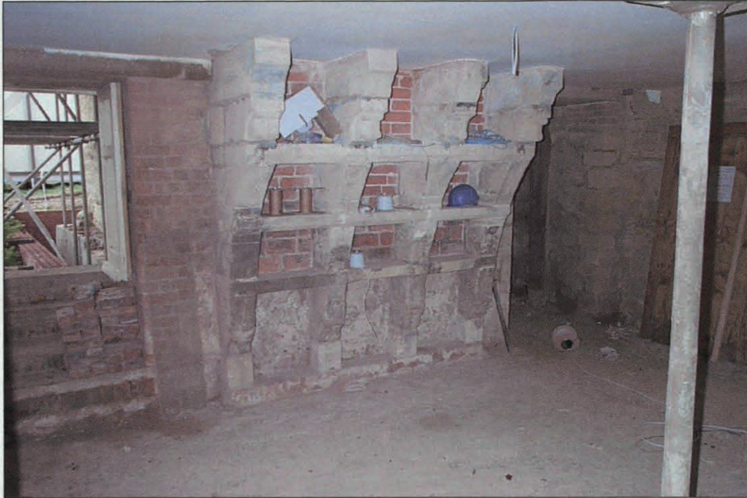
Plate 3: Stone corbelling in cellar
