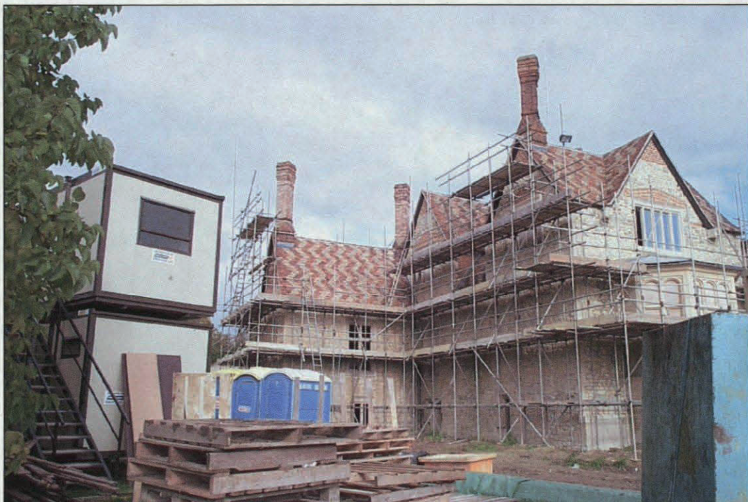
Plate 4: Dinton Hall, west wing from south-west
