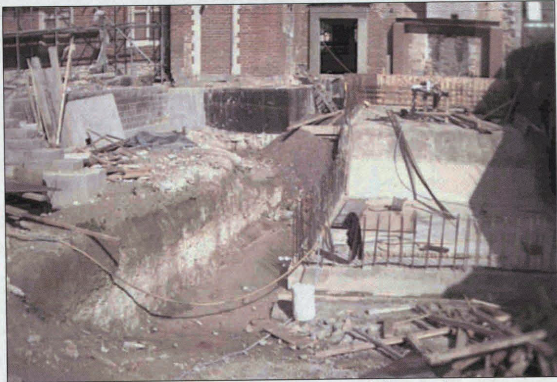
Plate 7: Excavation for swimming pool, from south.
