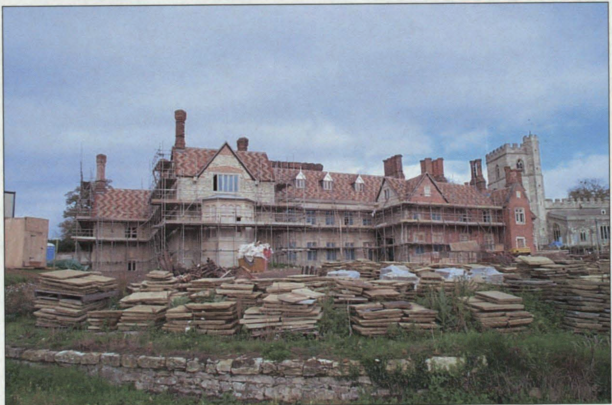
Plate 1: Dinton Hall, south frontage.
