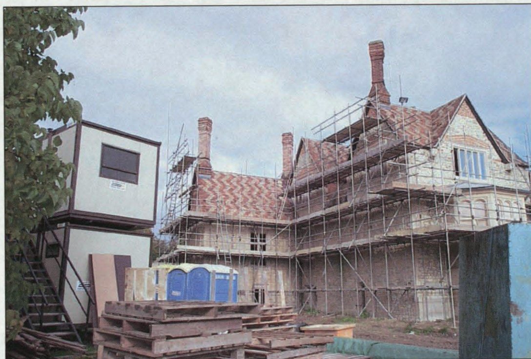
Plate 4: Dinton Hall, west wing from south-west
