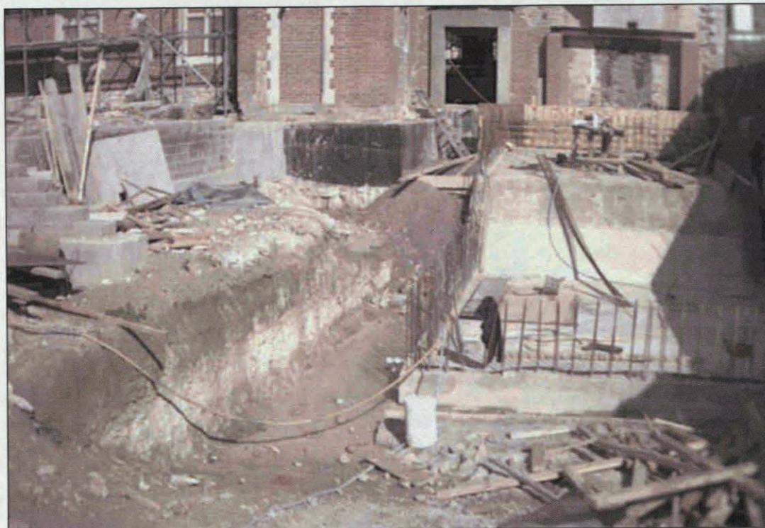
Plate 7: Excavation for swimming pool, from south.
